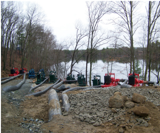
The March 2010 Culvert collapse work on Rt. 119. 1.7 million Gallons of water a day being pumped
