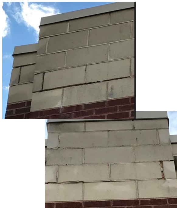
Failed mortar joints
