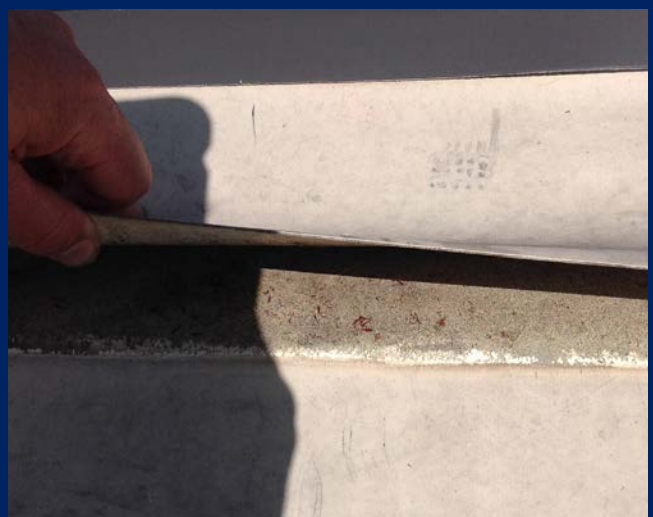
Evidence of water ponding, signs of aged flashings can be seen where membranes separate, or "pull back". (Classroom Wing - Roof 5)
