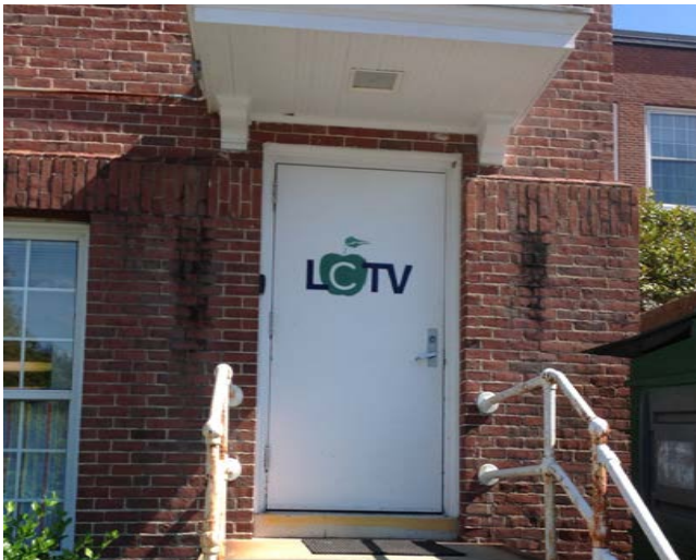
Evidence of staining/soiling on either side of door. (Multi-Use Wing - Parking Lot Side)
