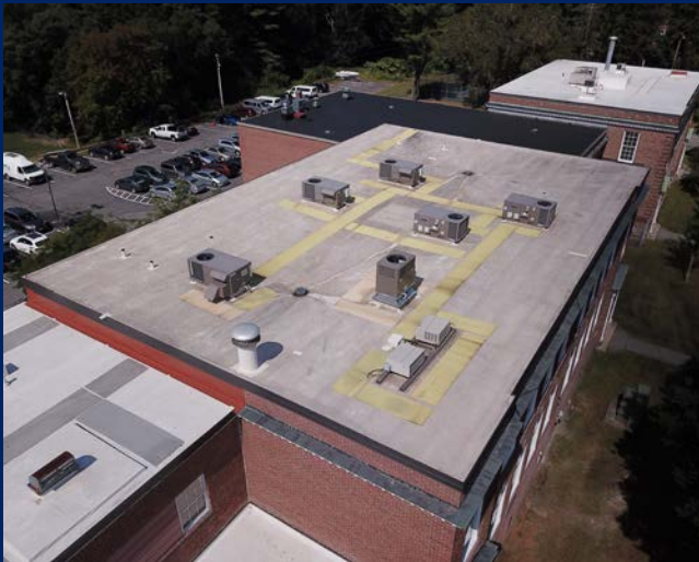
Overall discoloration of roof. (Classroom Wing - Roof 5)
