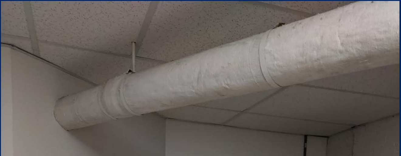
Pipe TSI - Confirmed ACM (Multi-Use Wing - Third Floor Storage Room)
