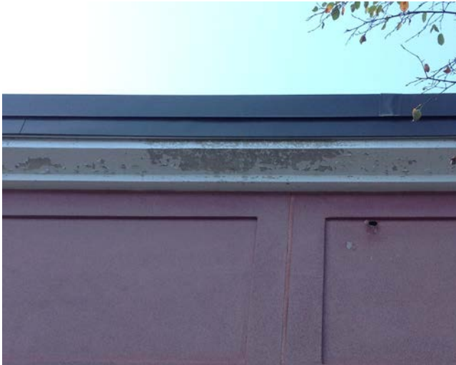
Observed peeled paint on trim board. (Library Wing - Shattuck Street Side)
