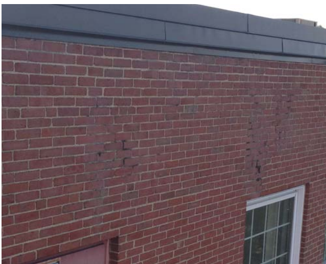
Evidence of staining/soiling on third floor, most likely from water damage. (Classroom Wing - Parking Lot Side)
