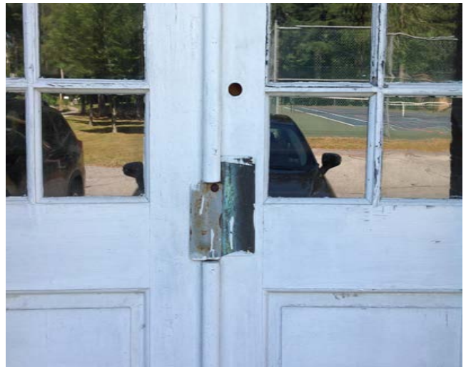
Evidence of damaged & deteriorated paint finish. (Office Wing - Tennis Court Side)
