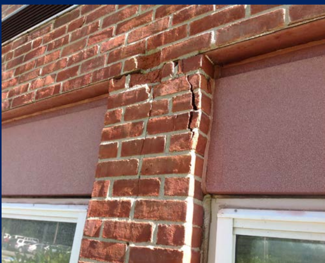
Evidence of brick spalling, most likely from uneven compression and/or water damage. (Library Wing - Parking Lot Side)
