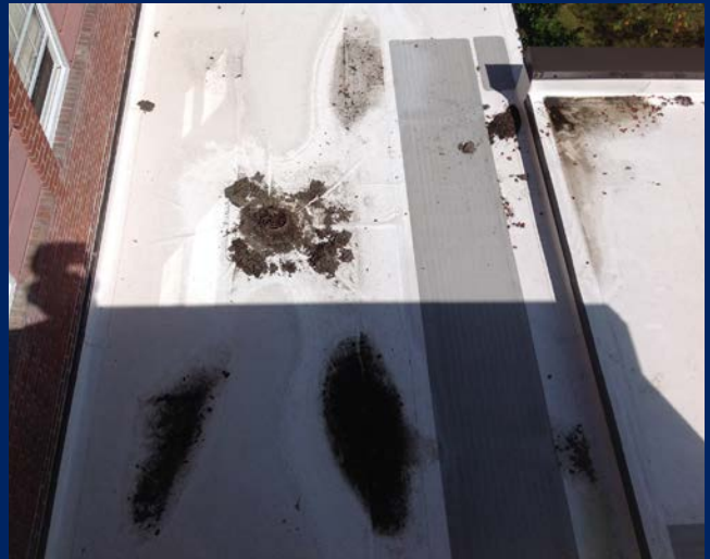
Evidence of ponding of water and debris near roof drain. (Library Wing - Roofs 3 & 4)
