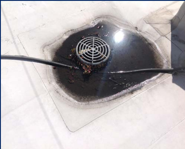
Ponding on roofing at roof drain. (Office Wing - Roof 8)
