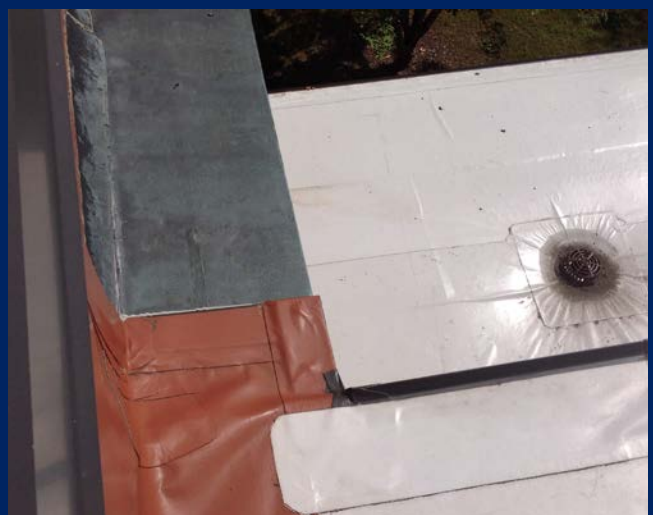
Gap in base flashing. (Library Wing - Roof 2)
