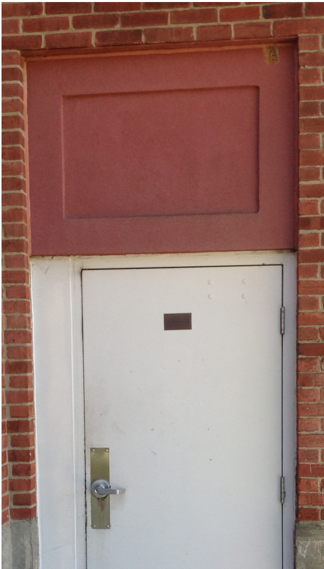
Evidence of damage to EIFS above conference room door. (Library Wing - Parking Lot Side)
