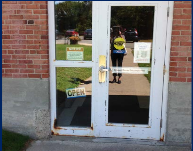
Evidence of damaged & deteriorated paint finish, and rotting (loss) of core material. (Library Wing - Parking Lot Side)
