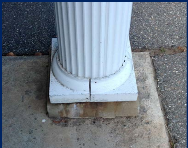
Evidence of cracking/separation of column trim. (Library Wing - Shattuck Street Side)
