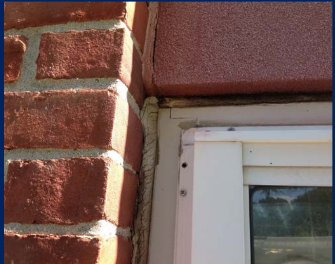
Evidence of cracked caulking at window opening. (Library Wing - Parking Lot Side)
