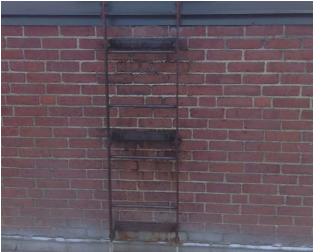
Visible rust and water damage behind access ladder on roof. (Multi-Use Wing to Classroom Wing)
