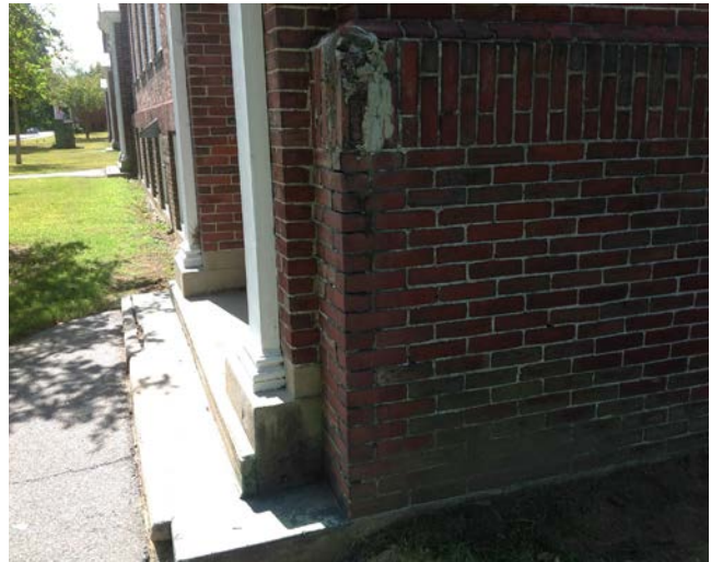
Evidence of attempted patch of corner with mortar and areas of missing mortar. (Office Wing - Shattuck Street Side)
