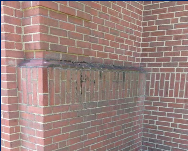
Evidence of staining/soiling, most likely from water damage. (Library Wing - Shattuck Street Side)
