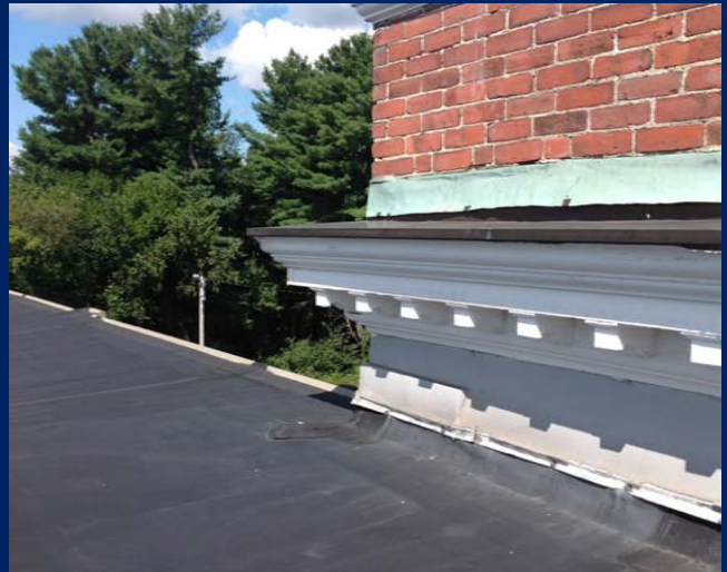
Observed staining/soiling on trim board. (Multi-Use Wing Roof to Office Wing Roof)
