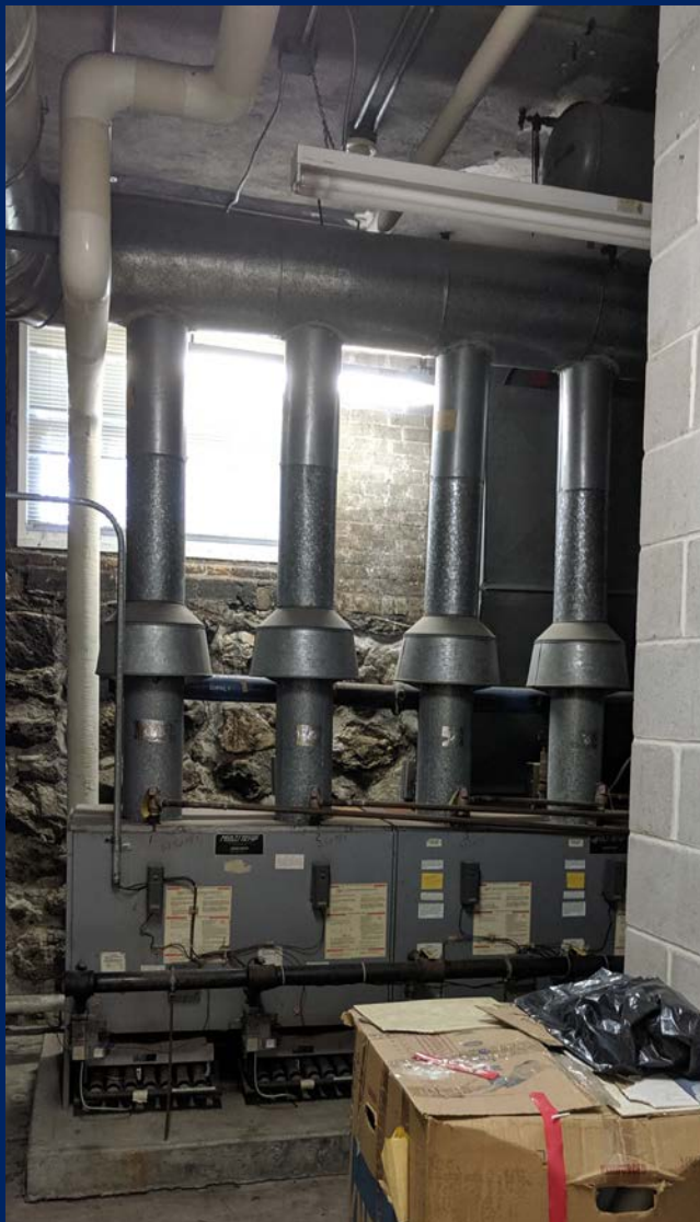
One of two boiler plants, both in need of replacement. (Office Wing - First Floor)
