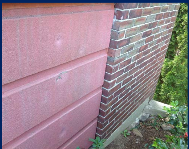
Evidence of damage to EIFS. (Multi-Use Wing - Parking Lot Side)
