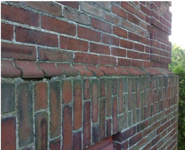
Evidence of staining/soiling, most likely from water damage. (Office Wing - Tennis Court Side)
