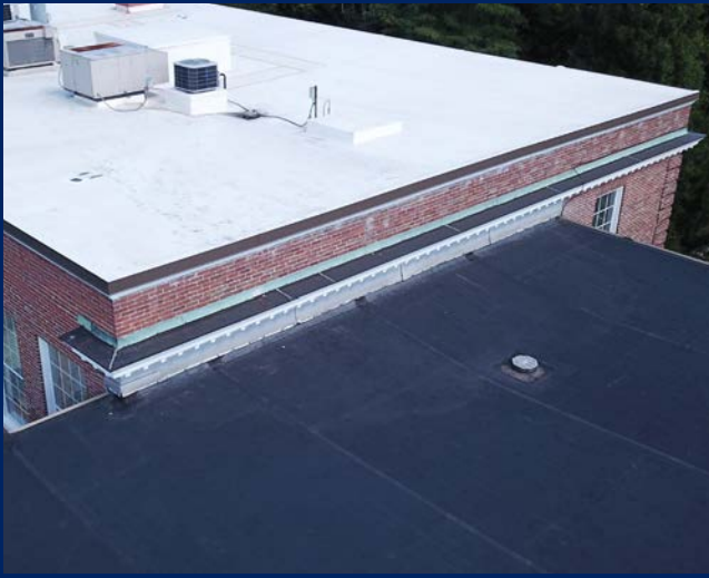
Discoloration of roof shows evidence of ponding on roofing near roof drain. (Multi-Use Wing - Roof 6)
