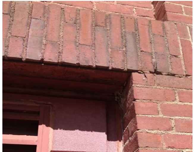
Evidence of staining/soiling and areas of missing mortar. (Multi-Use Wing - Parking Lot Side)
