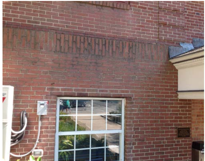
Evidence of staining/soiling near main entrance, most likely from water damage. (Classroom Wing - Parking Lot Side)
