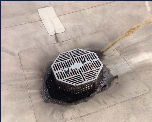
Evidence of ponding of water near roof drain. (Classroom Wing - Roof 5)
