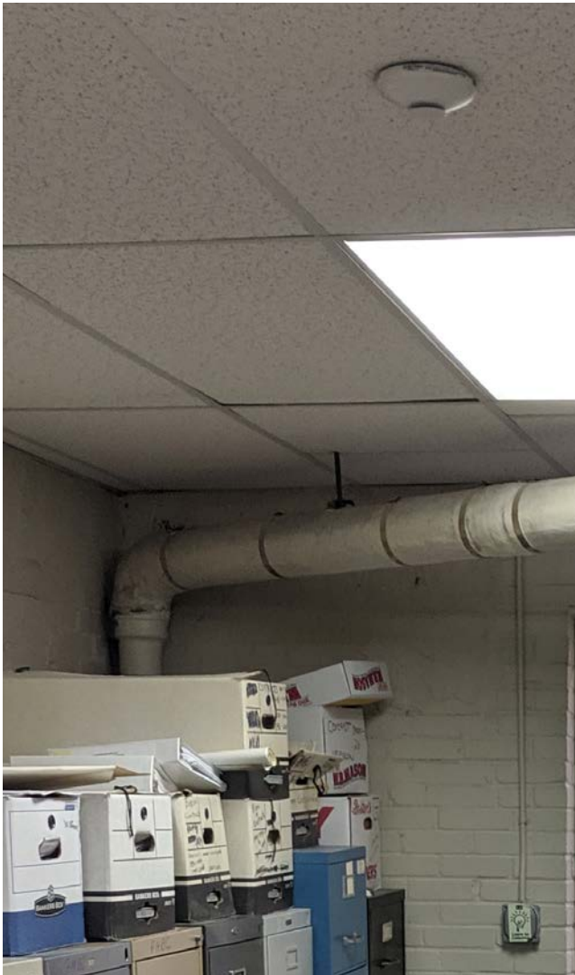
Pipe TSI - Confirmed ACM (Multi-Use Wing - Third Floor Storage Room)
