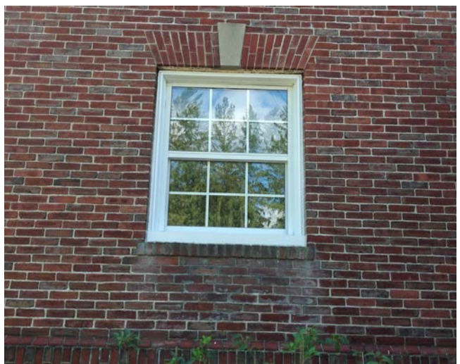
Evidence of staining/soiling at window sill. (Office Wing - Tennis Court Side)
