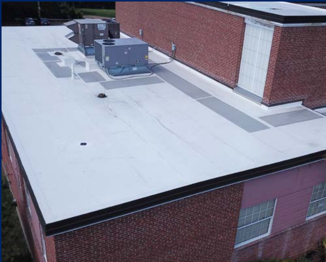
Evidence of rippling at roof membrane seams which could be indicative of water leakage. (Library Wing - Roof 1)
