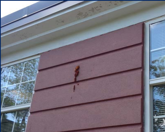
Damage from nesting birds that has been reactively filled with spray foam that does not match finish of Dryvit. (Library Wing - Shattuck Street Side)
