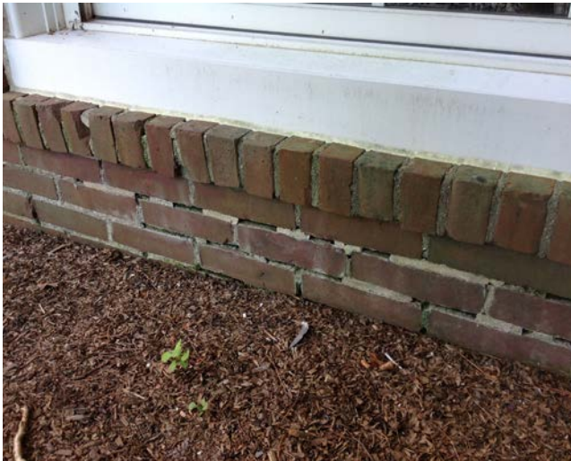
Evidence of staining/soiling and mortar erosion at window sill, most likely from water damage. (Office Wing - Parking Lot Side)
