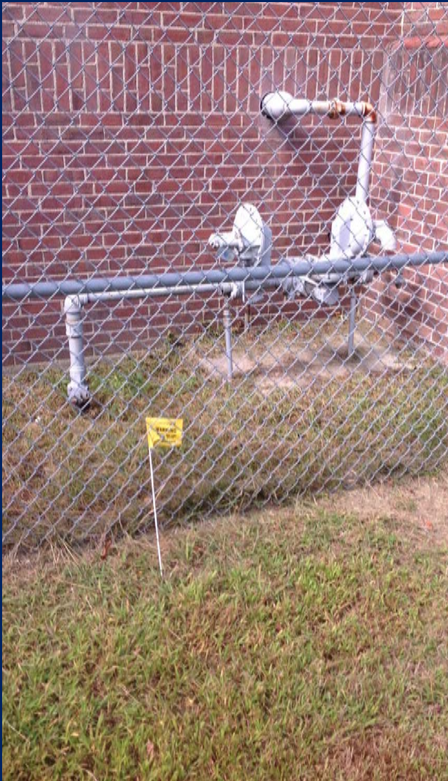
Water meter and check valve. (Multi-Use Wing - Shattuck Street Side)
