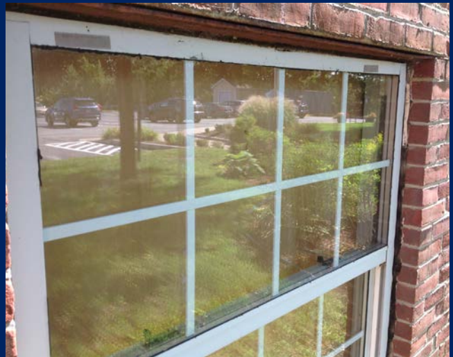
Evidence of cracked caulking and discoloration at window opening. (Classroom Wing - Parking Lot Side)
