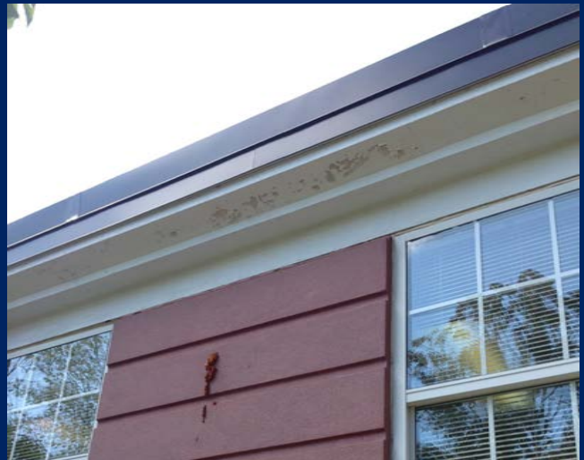
Observed peeled paint on trim board. (Library Wing - Shattuck Street Side)
