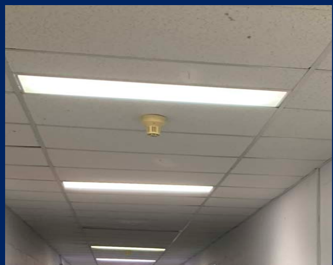
Typical 2' x 4' recessed fluorescent lighting fixtures throughout corridors and offices. (Classroom Wing - First Floor)
