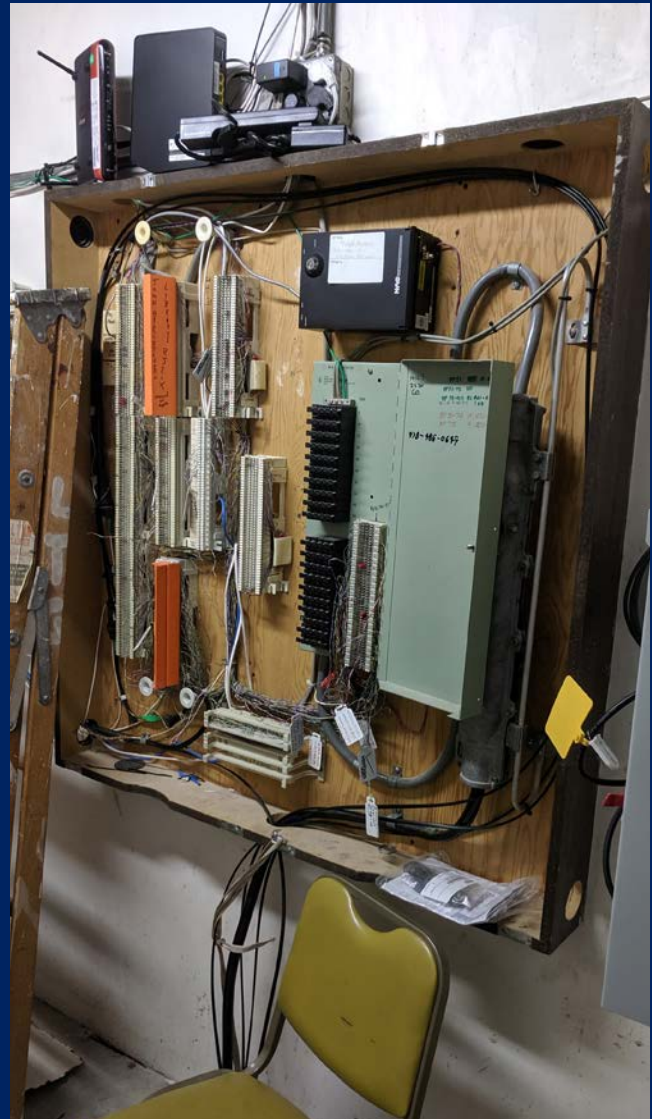
Main tele/data panel. (Classroom Wing - First Floor)
