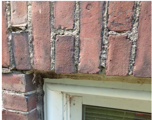
Evidence of eroded mortar joint near window opening. (Office Wing - Shattuck Street Side)
