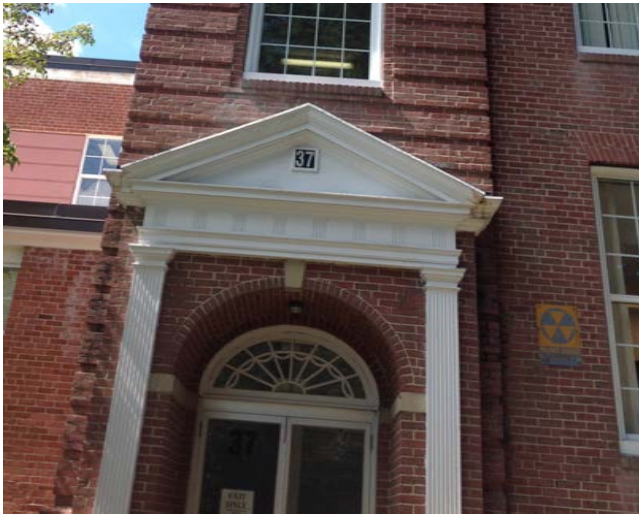
Evidence of water damage on pediment trim. (Classroom Wing - Shattuck Street Side)
