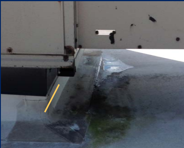
Evidence of ponding of water near mechanical unit. Gap in base flashing. (Office Wing - Roof 8)
