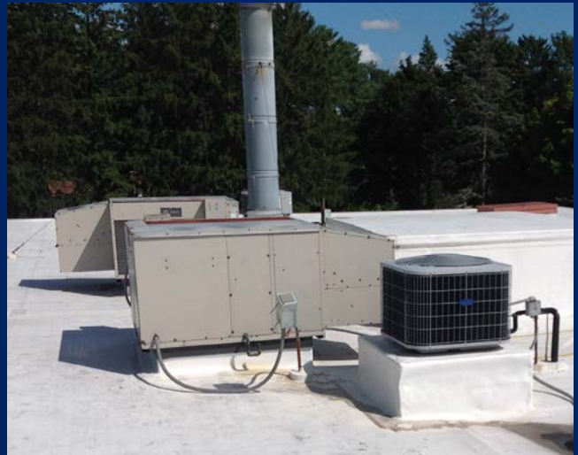
One of a few older rooftop air handling unit (RTUs) located on the Multi-Use & Office roofs. (Office Wing - Roof 8)
