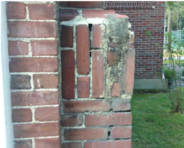
Evidence of attempted patch of corner with mortar and areas of missing mortar. (Office Wing - Shattuck Street Side)
