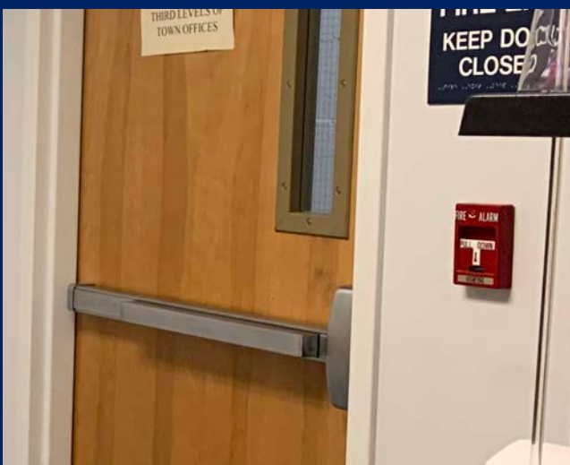
Typical fire alarm pull located throughout the building. (Library Wing - First Floor)
