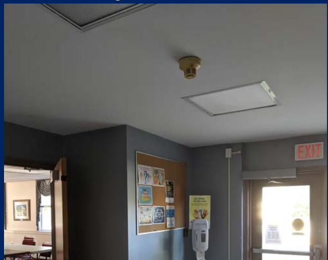
Typical painted GWB ceiling condition. (Library Wing - First Floor)
