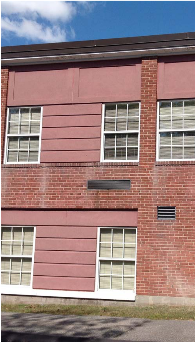
Evidence of staining/soiling at window sills; typical at all window openings on all buildings. (Library Wing - Parking Lot Side)
