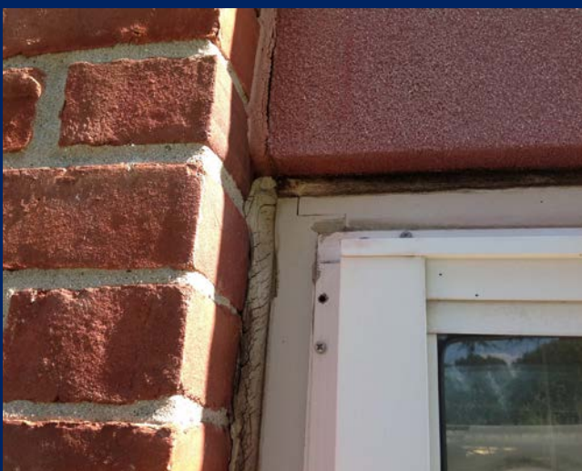
Evidence of cracked sealant between EIFS, masonry, and window. (Library Wing - Parking Lot Side)
