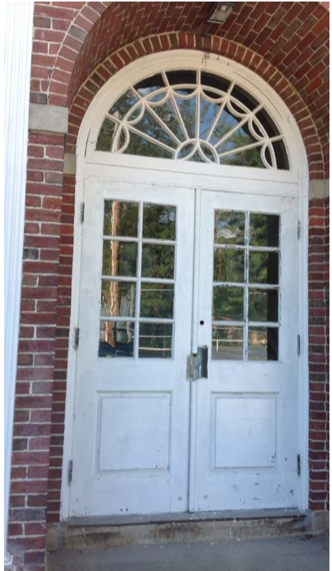
Observed peeled paint on trim board. (Office Wing - Tennis Court Side)
