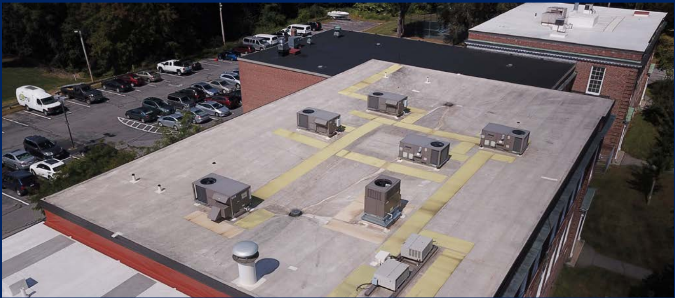
Numerous relatively new rooftop air handling unit (RTUs) located on the Classroom roof. (Classroom Wing - Roof 5)
