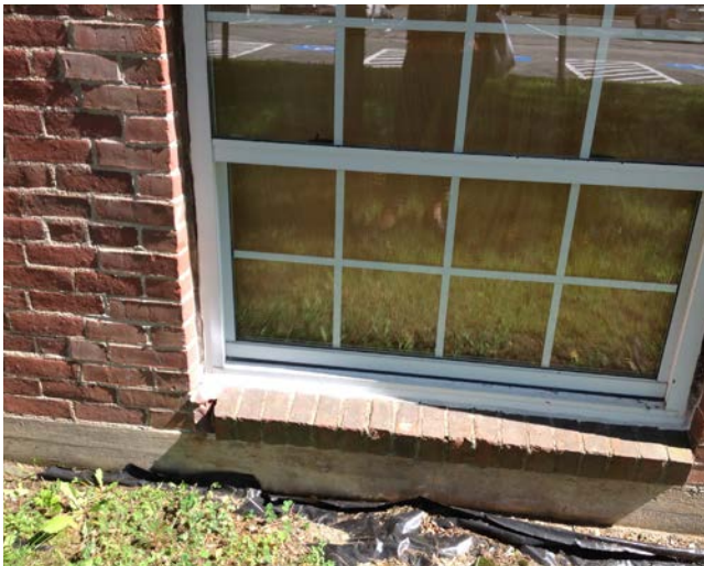
Evidence of brick delaminating and eroding mortar at window sill. (Classroom Wing - Parking Lot Side)
