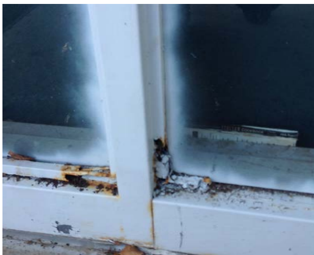
Close-up at of aluminum sidelight sill at library main entrance. (Library Wing - Shattuck Street Side)
