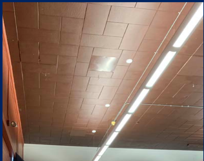
Old glued acoustical ceiling system, painted finish may compromise performance in LCTV Studio. (Multi-Use Wing - Second Floor)
