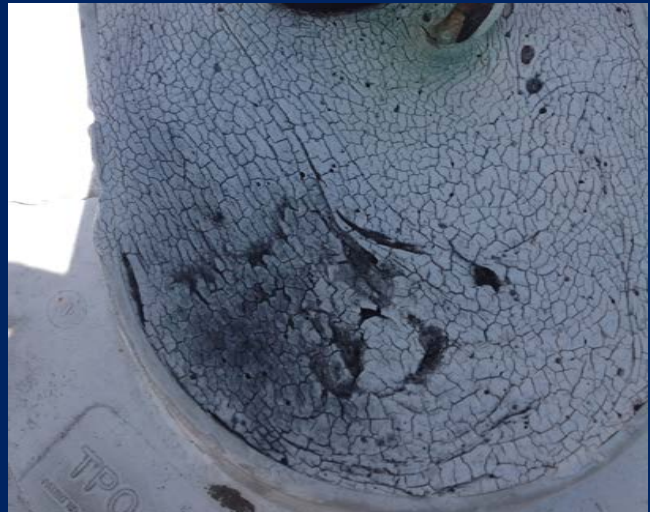
Evidence of cracked roofing membrane, due to moisture damage / ponding of water. (Office Wing - Roof 8)
