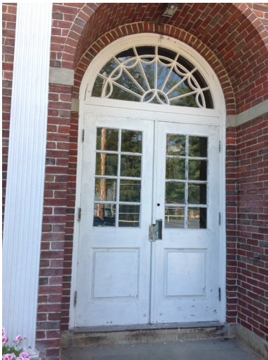
Evidence of damaged & deteriorated paint finish. (Office Wing - Tennis Court Side)
