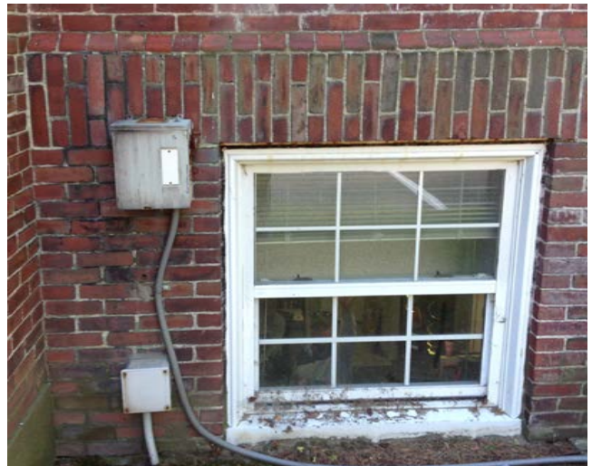
Evidence of staining/soiling near window opening. (Office Wing - Tennis Court Side)
