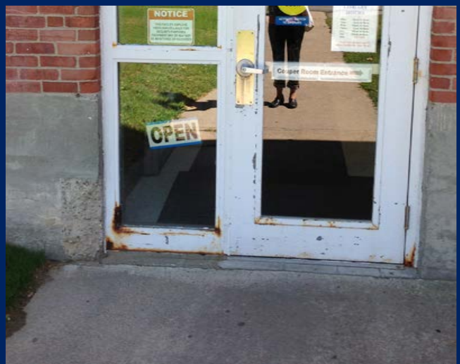
Visible deterioration of concrete, exposing the aggregate. (Library Wing - Parking Lot Side)
