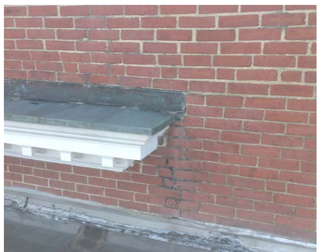
Evidence of staining/soiling and mortar erosion, most likely from water damage. (Multi-Use Wing Roof to Office Wing Roof)
