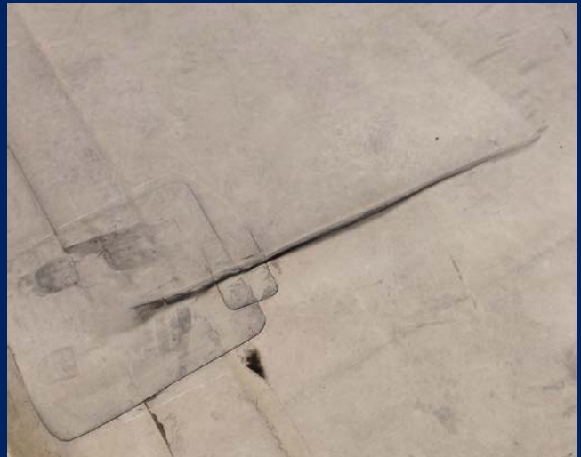
Wrinkled membrane poses a tripping hazard. (Classroom Wing - Roof 5)
