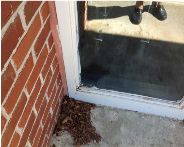
Evidence of damaged & deteriorated paint finish, and rotting (loss) of core material. (Office Wing - Parking Lot Side)
