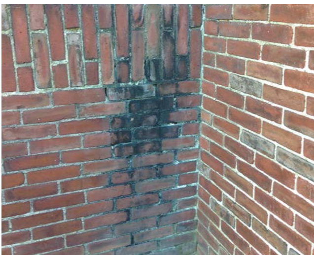
Evidence of staining/soiling, most likely from water damage or fire. (Office Wing - Tennis Court Side)
