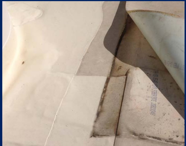
Separation of an already repaired joint (via applied darker coating) occurring in mansard wall. (Classroom Wing - Roof 5)
