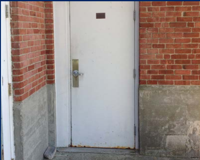
Evidence of rust/ deterioration exterior hollow metal door. (Library Wing - Parking Lot Side)
