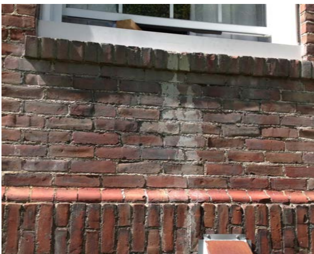
Evidence of efflorescence near window opening. (Office Wing - Shattuck Street Side)
