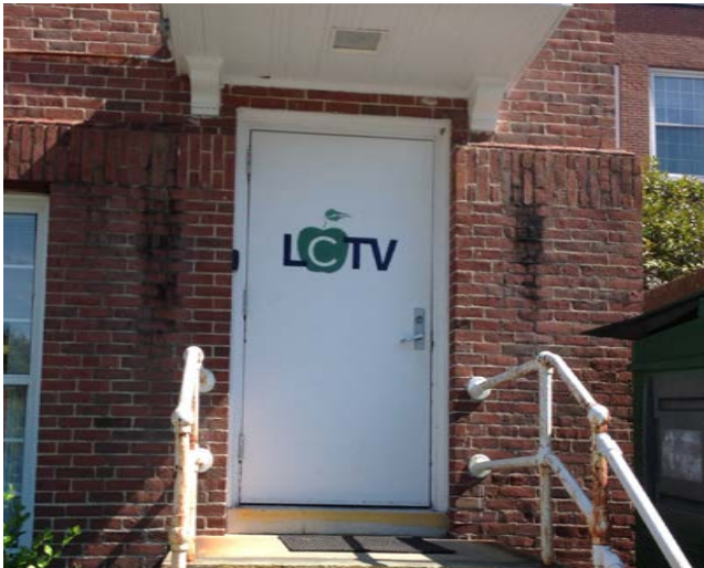
Exterior doors on the west facade showing signs of rust on the sills. (Multi-Use Wing - Parking Lot Side)
