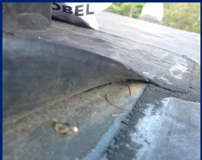
Evidence of water ponding, signs of aged flashings can be seen where membranes separate, or "pull back". (Multi-Use Wing - Roof 6)
