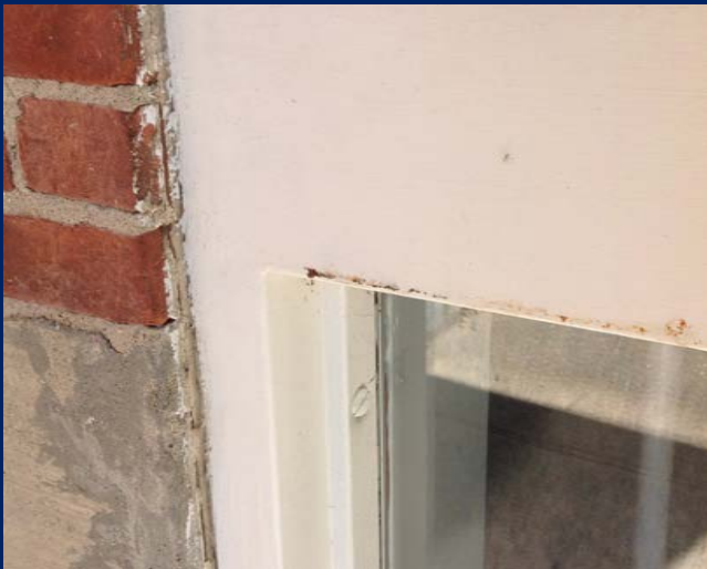
Evidence of minor rust and chipped paint on window frame. (Classroom Wing - Parking Lot Side)
