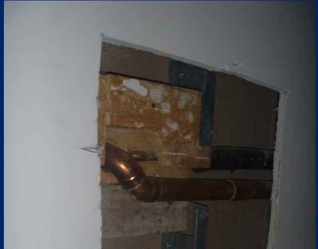
3" copper piping for domestic water distribution. (Library Wing)
