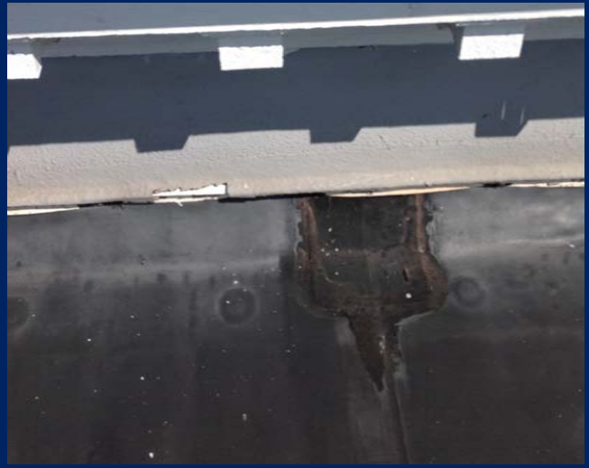
Evidence of damage to roofing where it meets the office wing. (Multi-Use Wing - Roof 6)
