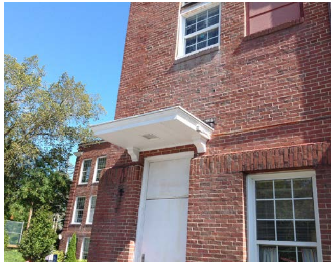
Exterior doors on the west facade showing signs of rust. (Multi-Use Wing - Parking Lot Side)
