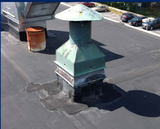
Evidence of a lot of patching previously done, making this a weak spot for water leakage in the future. (Multi-Use Wing - Roof 6)
