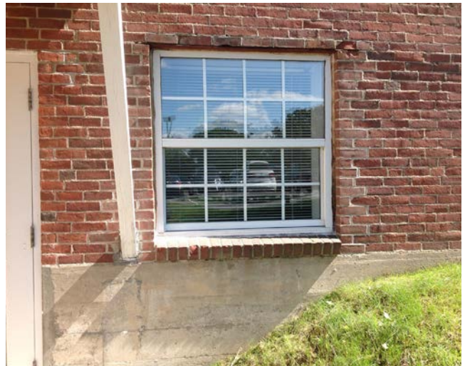
Evidence of brick delaminating and eroding mortar at window opening. (Classroom Wing - Parking Lot Side)
