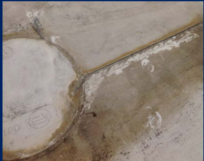
Evidence of moisture damage / ponding of water near roof seams. (Office Wing - Roof 8)
