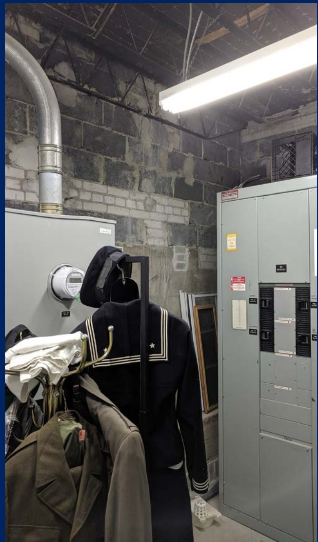
Electrical main and meters for each building. (Classroom Wing - First Floor)
