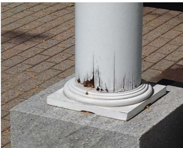
Evidence of cracking/missing wood on column trim. (Library Wing - Parking Lot Side)
