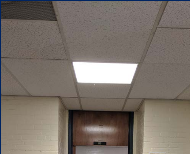
Typical 2x4 ACT ceiling condition in corridors. (Office Wing - First Floor)
