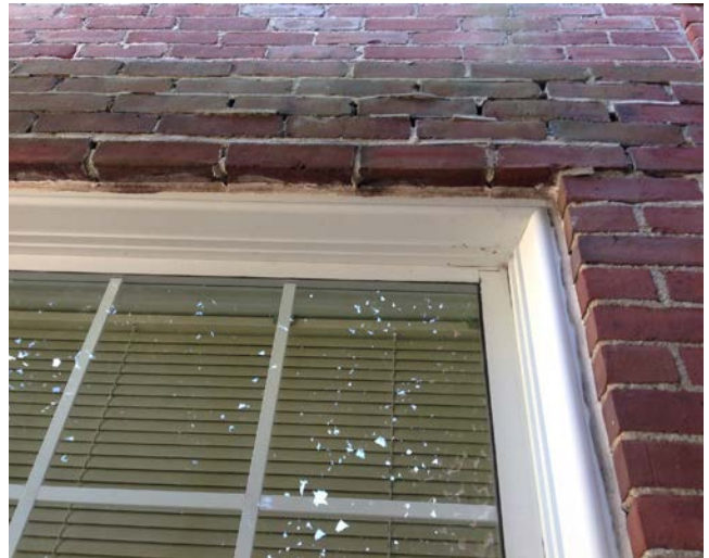
Evidence of staining/soiling at window header, most likely from water damage. (Office Wing - Parking Lot Side)
