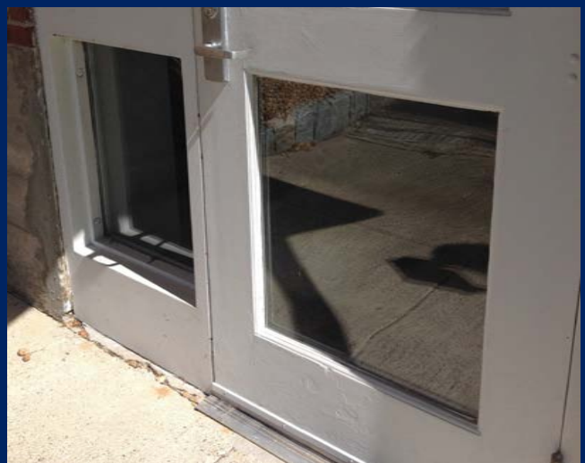
Evidence of damaged & deteriorated paint finish, and rotting core material. (Classroom Wing - Parking Lot Side)
