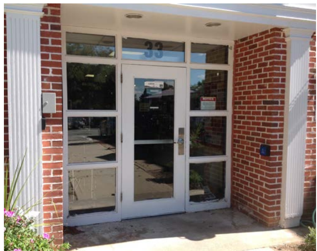
Evidence of damaged & deteriorated paint finish, and rotting (loss) of core material. (Office Wing - Parking Lot Side)
