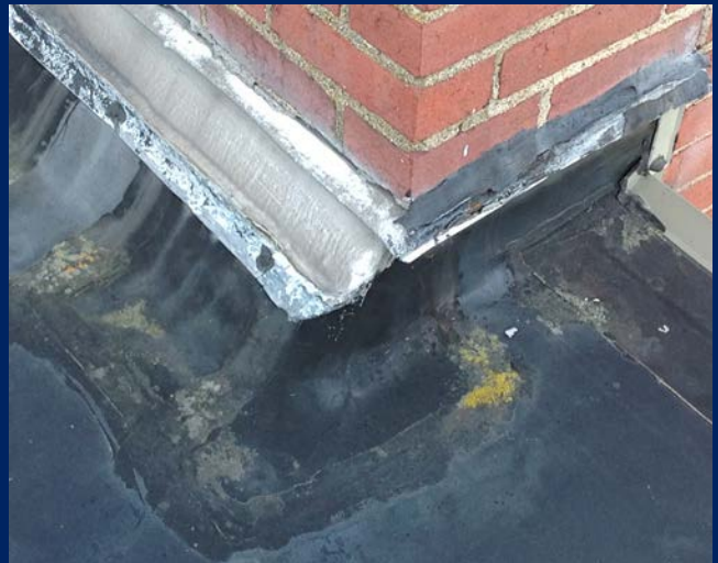
Organic growth around base flashing and gap in flashing near Classroom Wing. (Multi-Use Wing - Roof 6)
