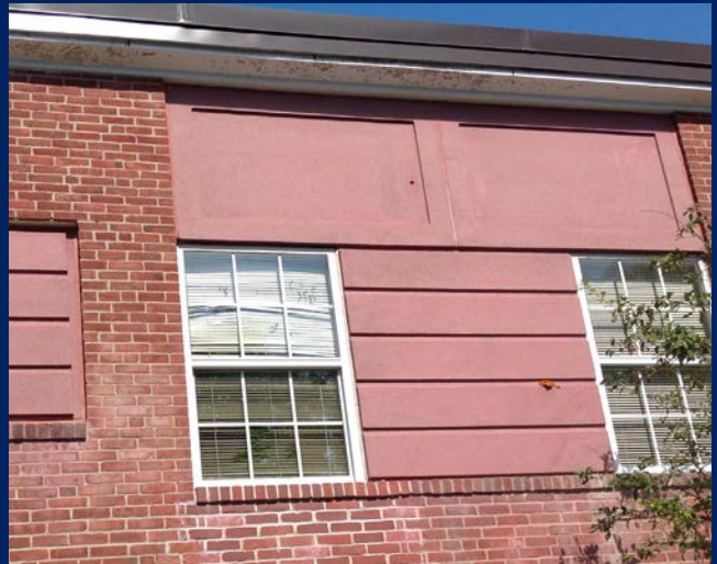
Damage from nesting birds that has been reactively filled with spray foam that does not match finish of Dryvit. (Library Wing - Parking Lot Side)
