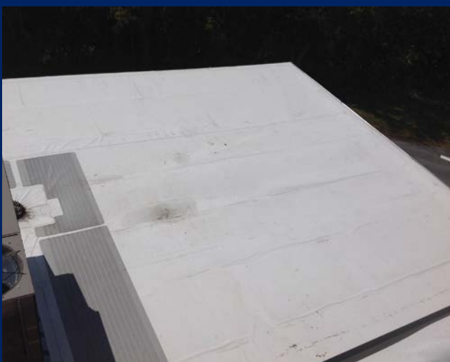
Evidence of rippling at roof membrane seams which could be indicative of water leakage. (Library Wing - Roof 2)
