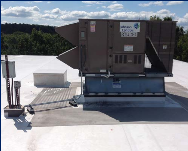
One of a few relatively new rooftop air handling unit (RTUs) located on the Library roofs. (Library Wing - Roof 2)
