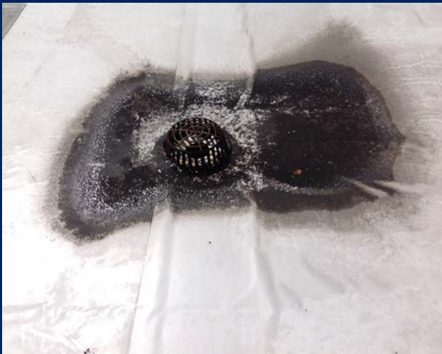
Evidence of ponding of water and debris near roof drain. (Library Wing - Roof 2)
