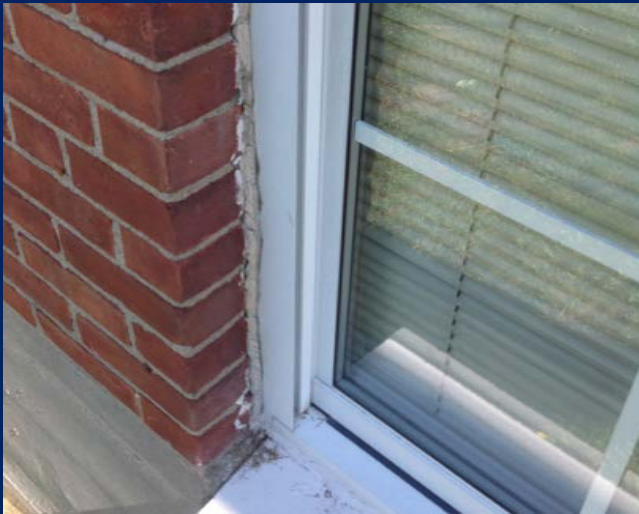
Evidence of cracked caulking at window opening. (Library Wing - Parking Lot Side)
