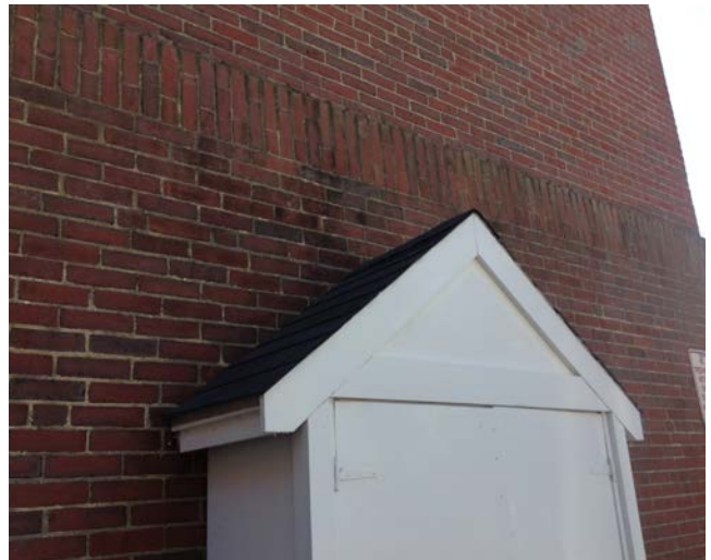
Evidence of staining/soiling, most likely from water damage. (Multi-Use Wing - Parking Lot Side)
