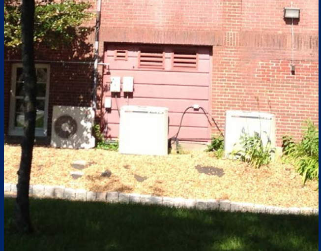
On grade split air handling units with condensing unit and compressor. (Multi-Use Wing - Parking Lot Side)
