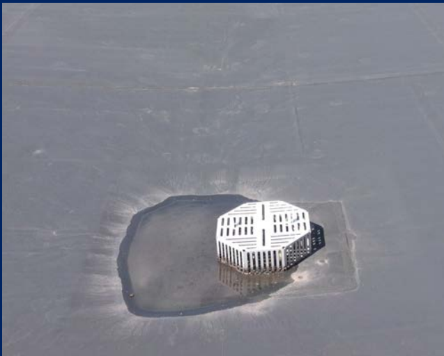
Evidence of ponding of water near roof drain. (Multi-Use Wing - Roof 6)
