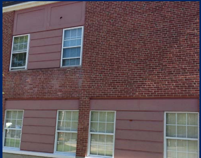
Evidence of mold/fungi growth on EIFS on ground level and damage on second floor. (Library Wing - Parking Lot Side)
