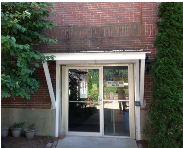
Evidence of damaged exterior door framing. (Multi-Use Wing - Parking Lot Side)
