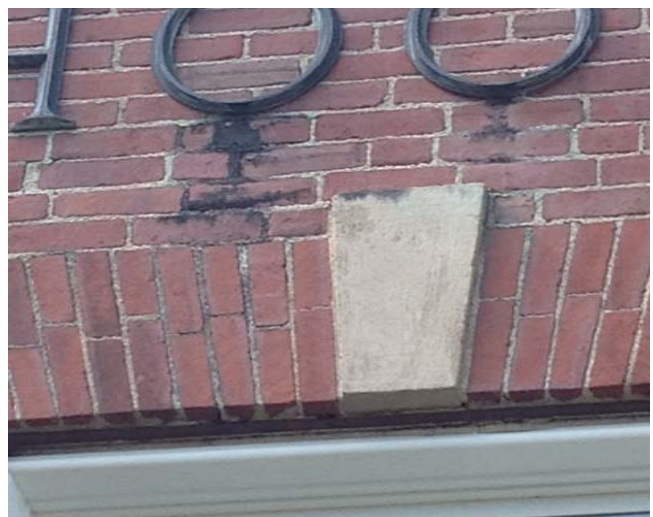
Evidence of staining/soiling, most likely from water damage. (Multi-Use Wing - Shattuck Street Side)
