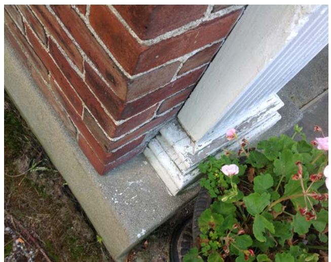
Observed peeled paint on trim board. (Office Wing - Tennis Court Side)
