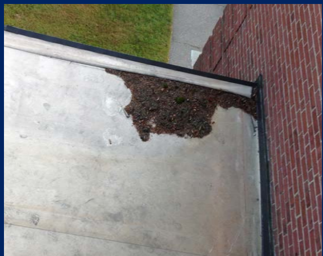
Organic growth around base flashing and gap in flashing. (Multi-Use Wing - Roof 7)
