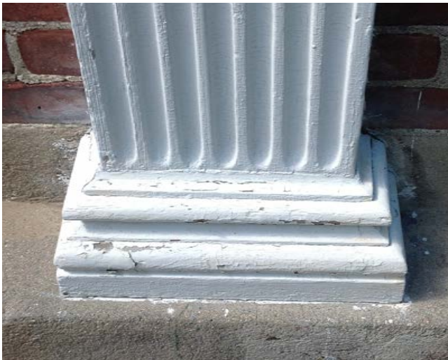
Observed peeled paint on trim board. (Office Wing - Shattuck Street Side)
