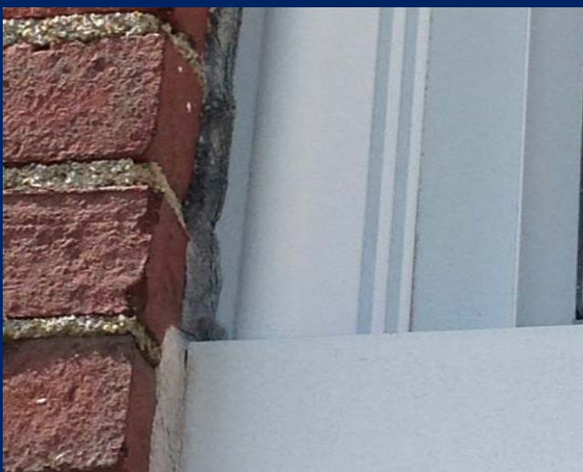
Evidence of cracked caulking and discoloration at window opening. (Multi-Use Wing - Parking Lot Side)
