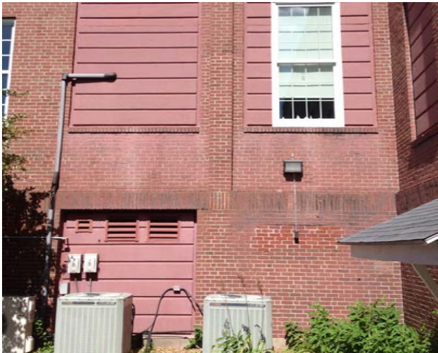
Evidence of staining/soiling, most likely from water damage. (Multi-Use Wing - Parking Lot Side)
