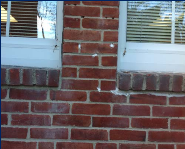
Evidence of staining/soiling at window sills. (Library Wing - Shattuck Street Side)
