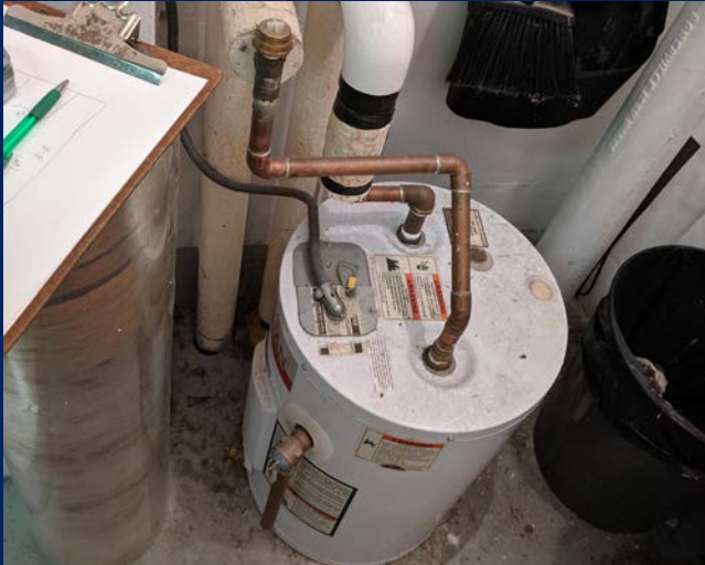
Small-capacity electric water heaters. (Classroom Wing - Second Floor)
