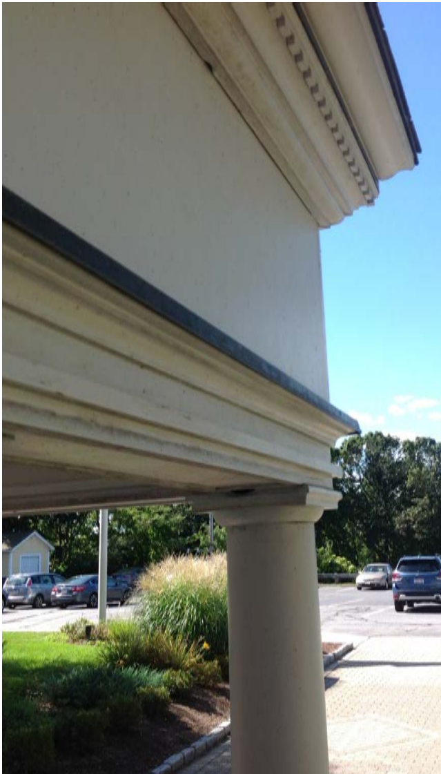
Observed staining/soiling on trim board. (Library Wing - Parking Lot Side)
