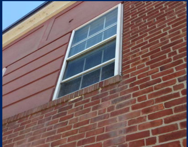
Evidence of staining/soiling at window sills; typical at all window openings on all buildings. (Library Wing - Parking Lot Side)
