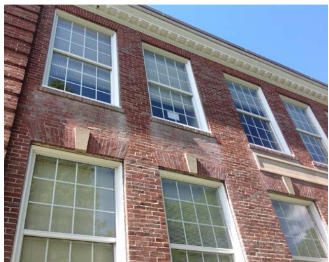
Evidence of staining/soiling at window sills. (Office Wing - Shattuck Street Side)
