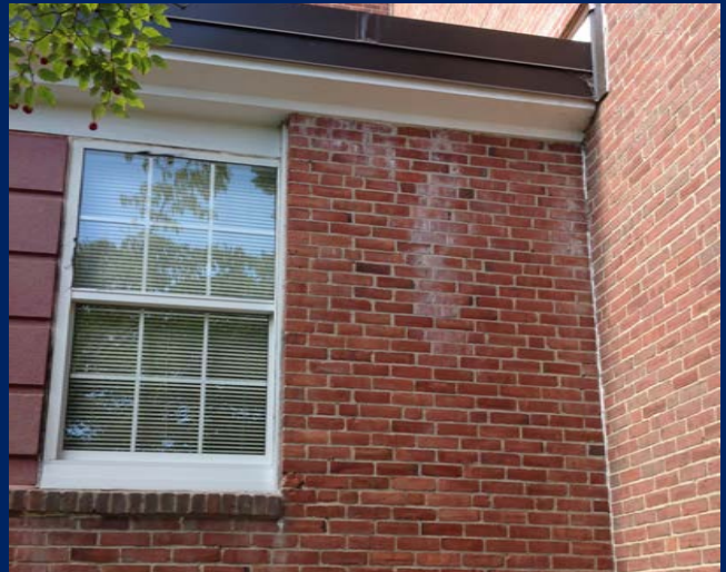
Evidence of efflorescence near window opening. (Library Wing - Shattuck Street Side)
