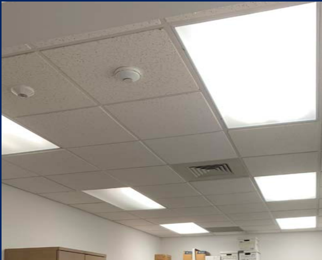
Typical office 2x2 ACT ceiling. (Classroom Wing - Second Floor)
