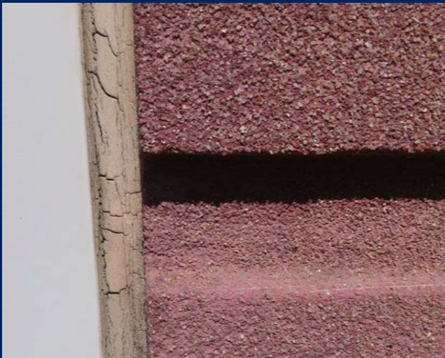
Evidence of eroding sealant between EIFS and window. (Library Wing - Parking Lot Side)
