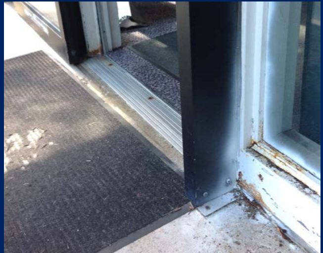
Evidence of damaged & deteriorated paint finish, and rotting (loss) of core material. (Library Wing - Shattuck Street Side)
