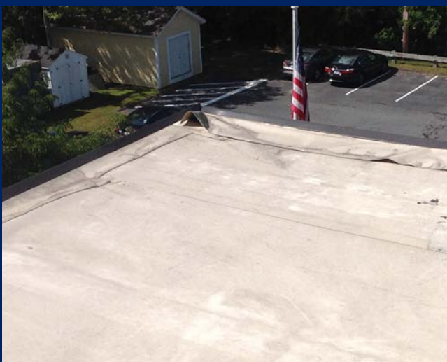
Evidence of water ponding, signs of aged flashings can be seen where membranes separate, or "pull back". (Classroom Wing- Roof 5)
