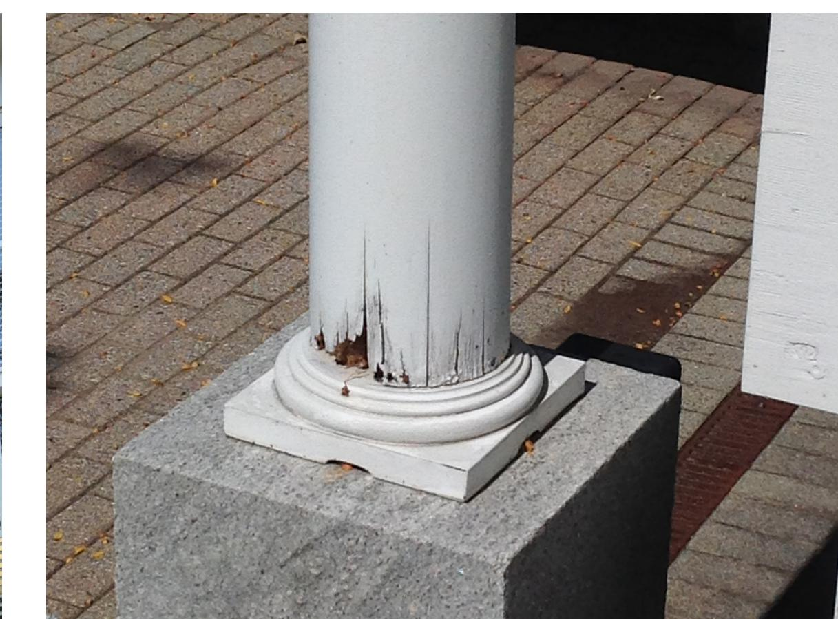
Evidence of cracking/missing wood on column trim. (Library Wing - Parking Lot Side)
