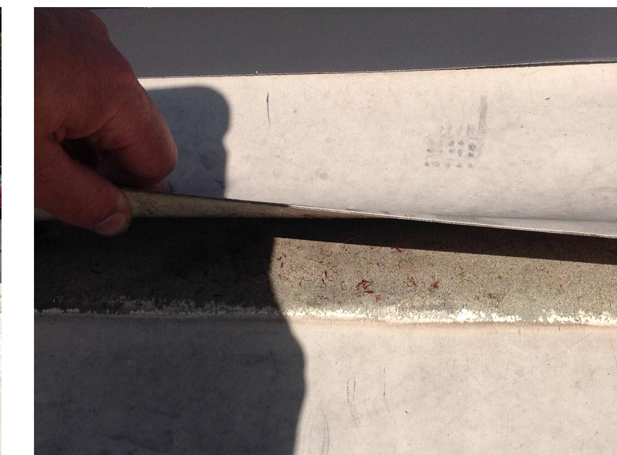
Evidence of water ponding, signs of aged flashings can be seen where membranes separate, or "pull back". (Classroom Wing - Roof 5)
