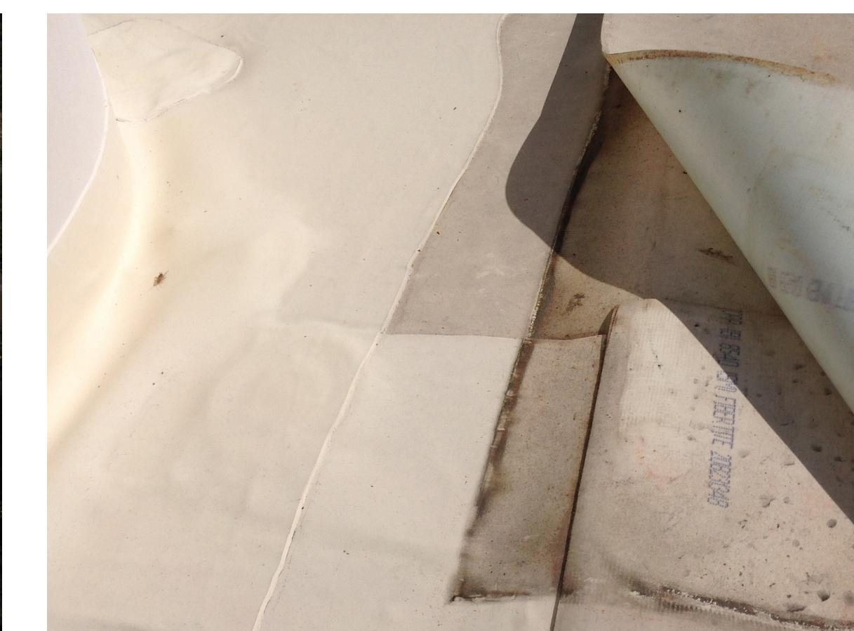
Separation of an already repaired joint (via applied darker coating) occurring in mansard wall. (Classroom Wing - Roof 5)
