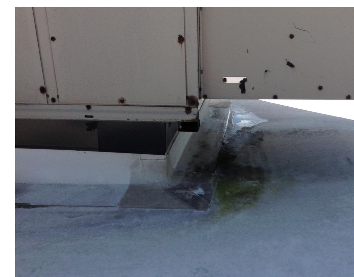
Evidence of ponding of water near mechanical unit. Gap in base flashing. (Office Wing - Roof 8)
