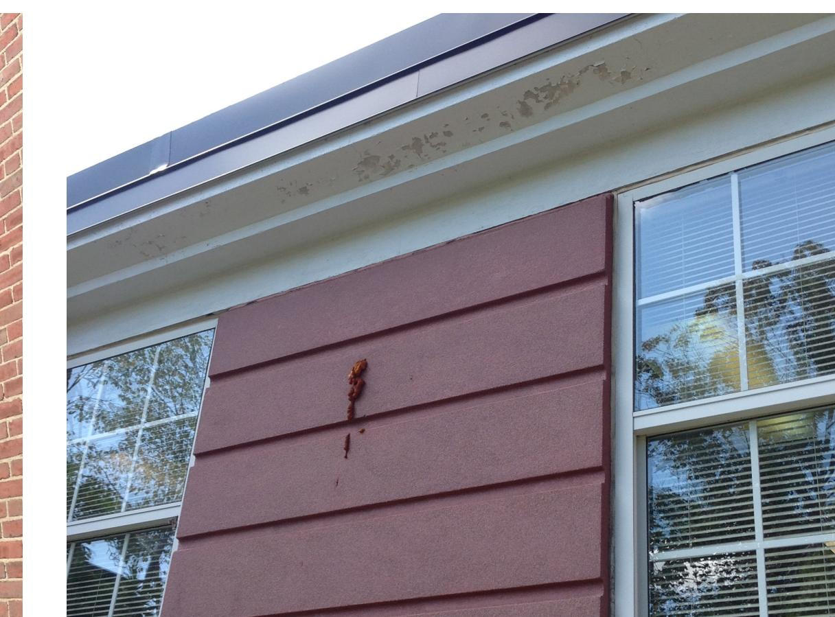
Damage from nesting birds that has been reactively filled with spray foam that does not match finish of Dryvit. (Library Wing - Shattuck Street Side)
