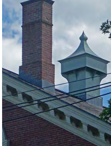
Ventilators, chimneys and other functional elements have long been used as an opportunity to add life and visual interest to the roofline of a building. These and other, more modern mechanical equipment, should be coordinated with the design of the whole structure, or screened from view.
