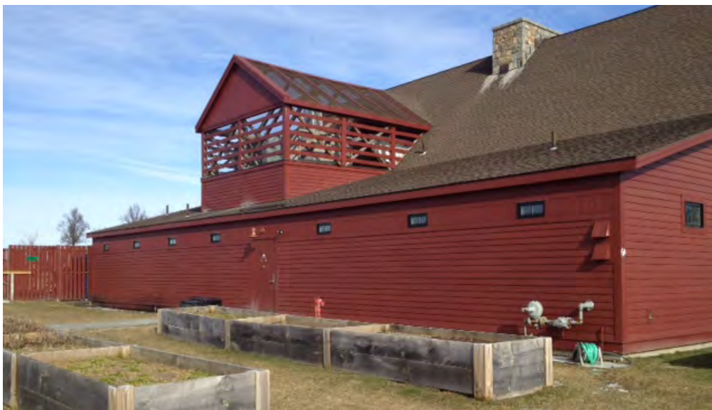
Modern rooftop mechanical equipment should be placed in an area that is not visible from the surrounding area or surrounded by architectural elements that fit the design of the building.
