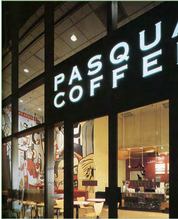
Individually mounted internally illuminated letters. Provide matte finish translucent vinyl film on face of letter.
