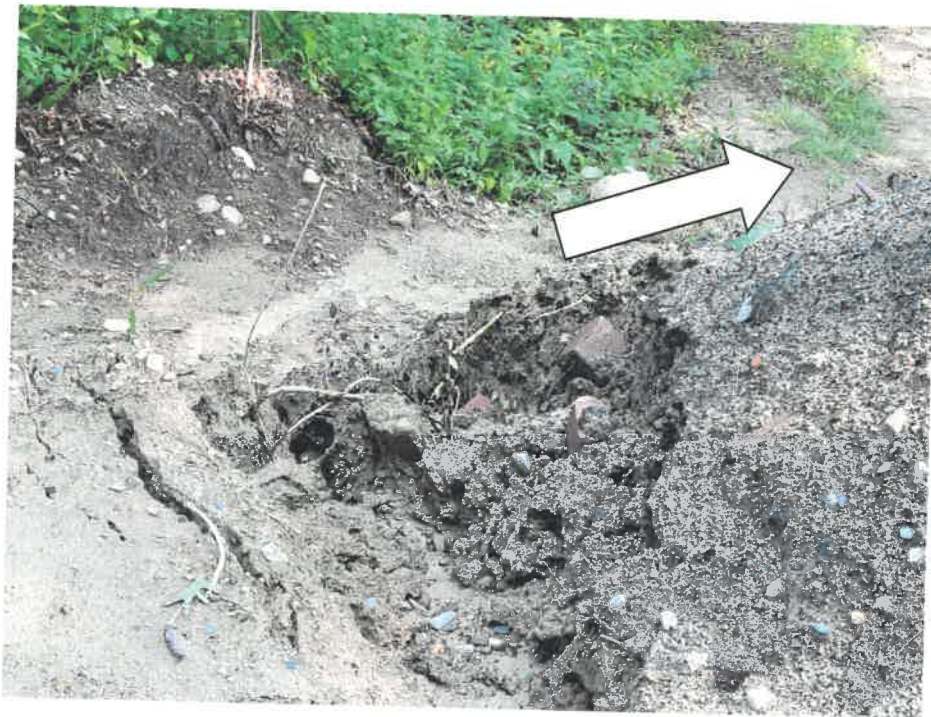
Photo 2. July 17, 2023. Close up of gully showing bricks etc in fill. Arrow shows siltation down the hill
