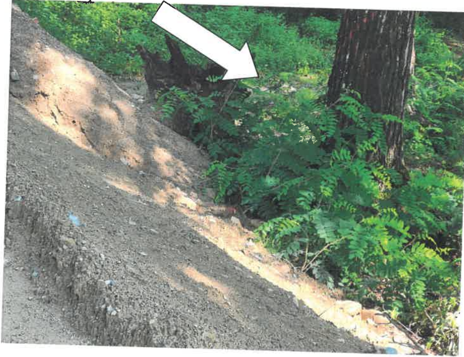
Photo 4. July 17, 2023. Heavy erosion going down hill. Tree trunk shown is part of 14"DEC and 18"DEC shown on the plans
