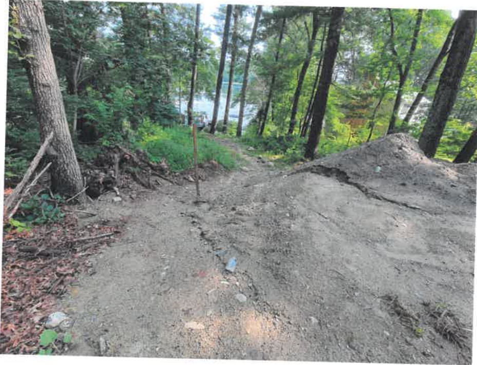
Photo 2. July 17, 2023. Close up of gully showing bricks etc in fill. Arrow shows siltation down the hill
