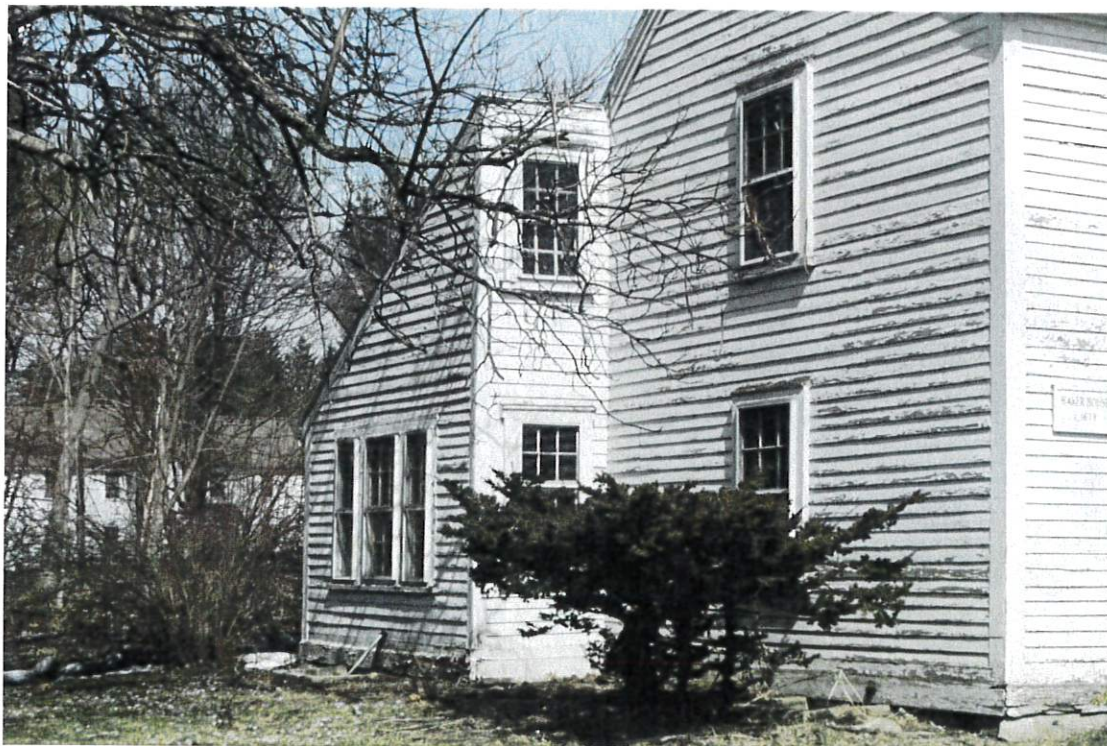
A detail of the Beverly jog on the west elevation of the Benjamin Kimball House.
