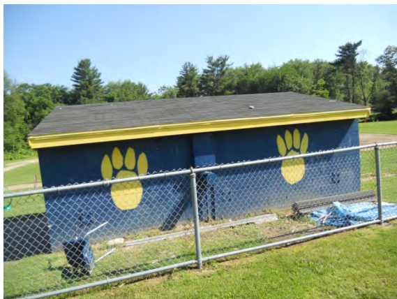
Photo #47: Rear and roof of dugout
