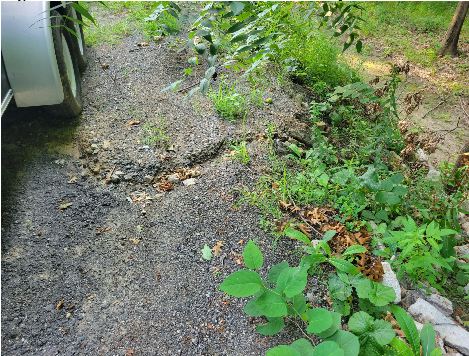
Figure 3. Some erosion in widened driveway. No sediment at toe of slope
